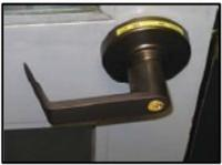
Outside knob locked or unlocked by key. Inside knob always unlocked.
