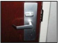
Push and turn button device. One motion in order to unlock and open the door.
