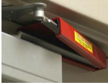
*Gatamate* enables teachers to lock the door quickly only using the foot from the inside.
